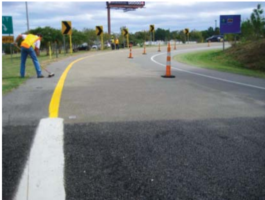
FIGURE 2: HFST at horizontal curve
