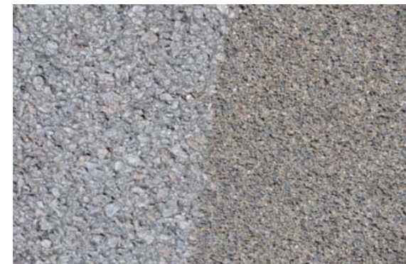
FIGURE 1: Open-grade surface course on the left and HFST on the right.
